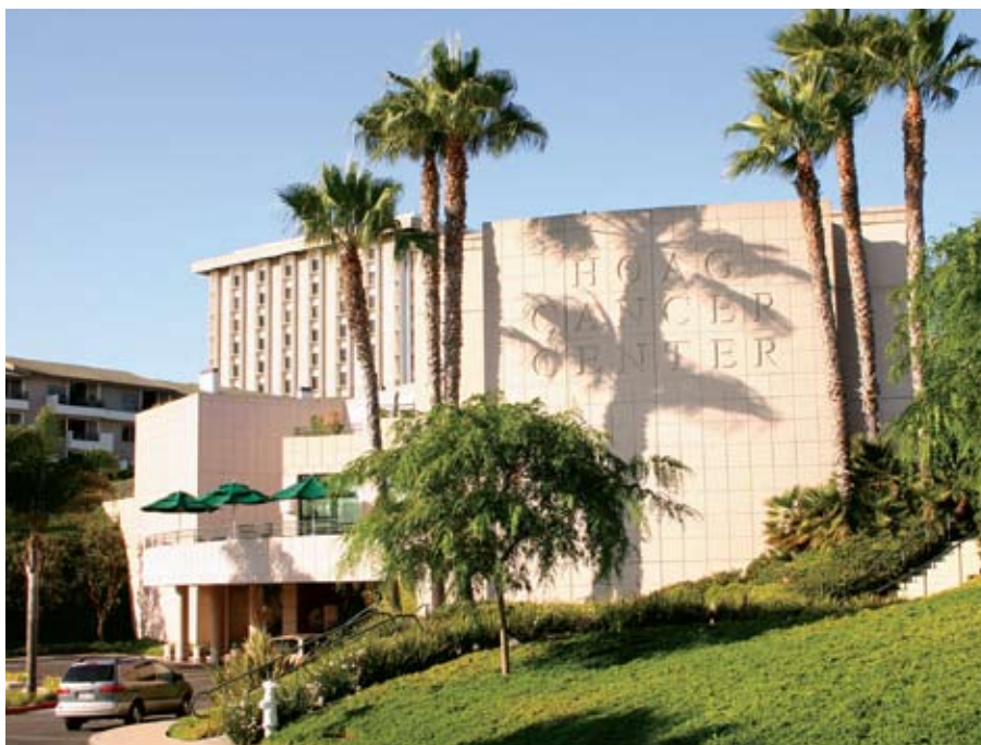
The Hoag Cancer Center in Newport Beach, California, includes a 65,000-square-foot, three-story facility that opened in 1991, and the oncology program of Hoag Hospital.
