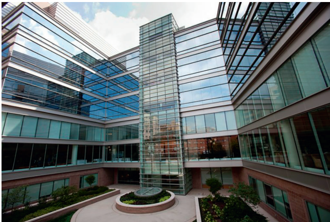
North Carolina Cancer Hospital, Chapel Hill, N.C.
