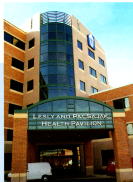
The new Lesly and Pat Sajak Pavilion at AAMC's Medical Park campus houses the Breast Center and the Anne Arundel diagnostic radiology facility.
